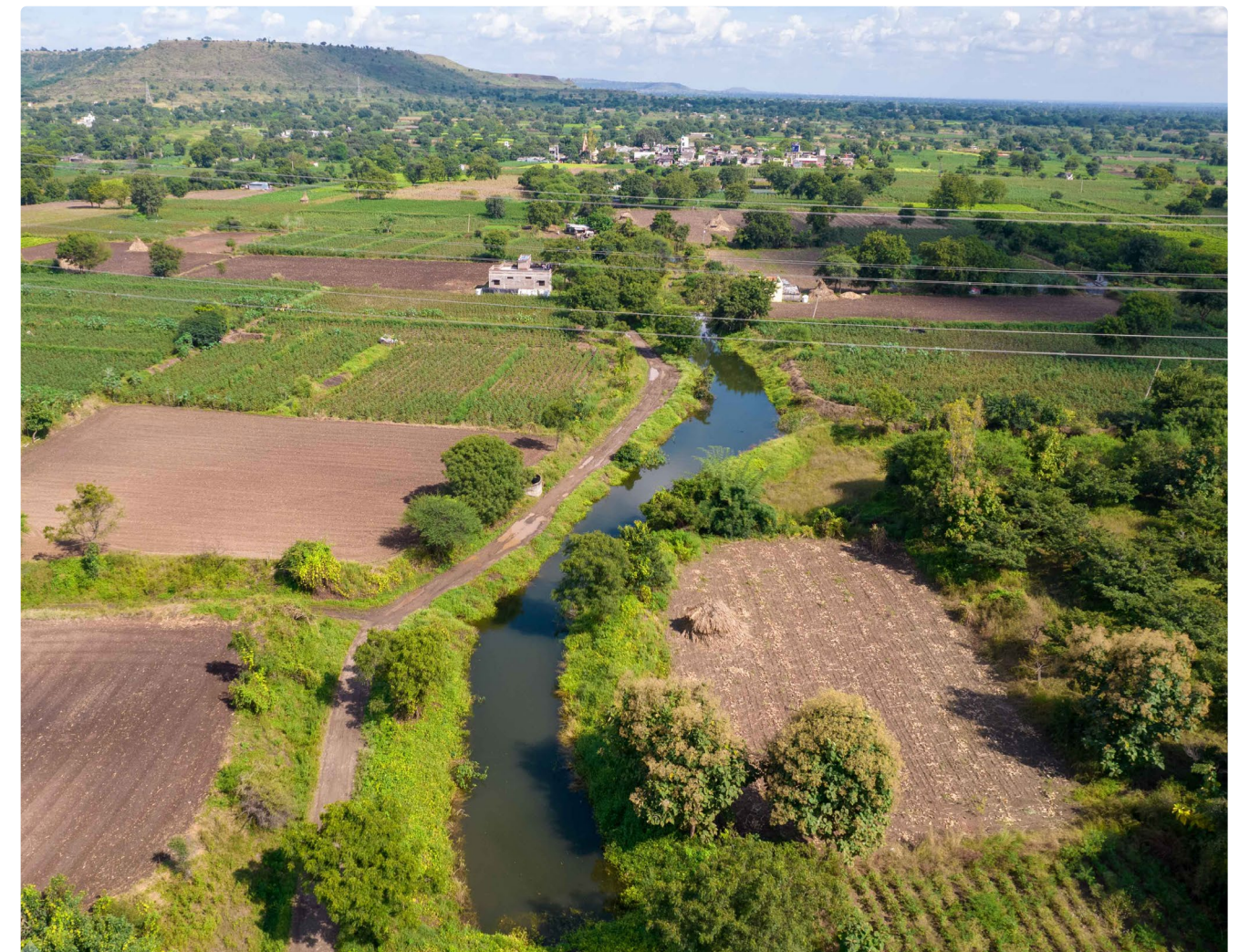
Canal deepened to increase water capacity
